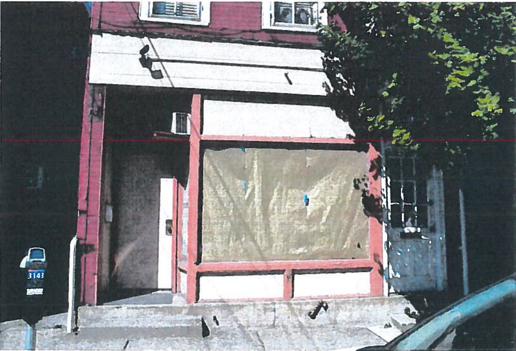
Figure 7. Overall view of storefront looking north.
