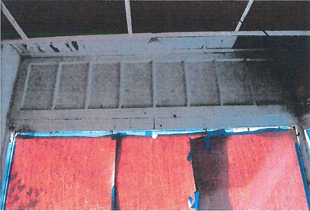
Figure 6. Close-up view of original painted-over transom at interior.
